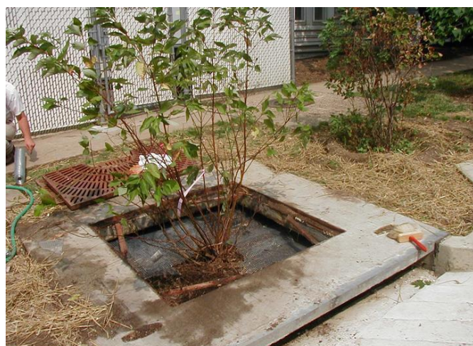
Figure B.2—Photograph of tree box filter.
