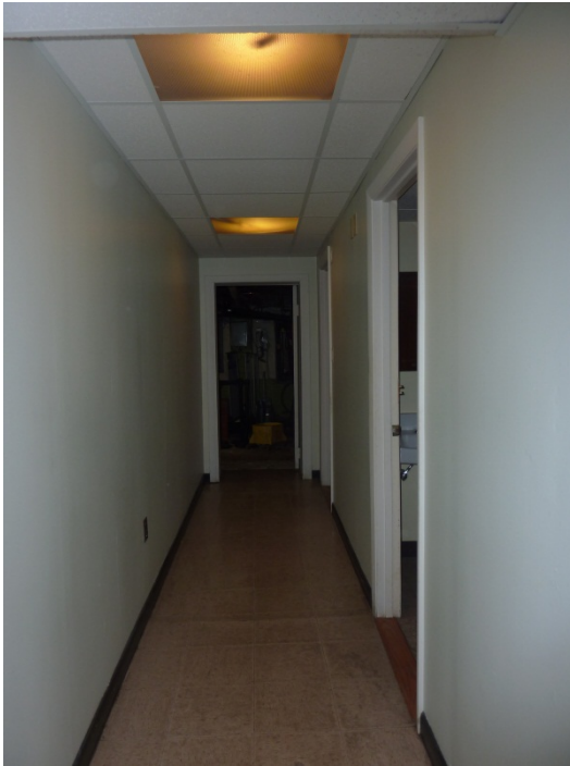
Vinyl tile in hallway at restrooms.
