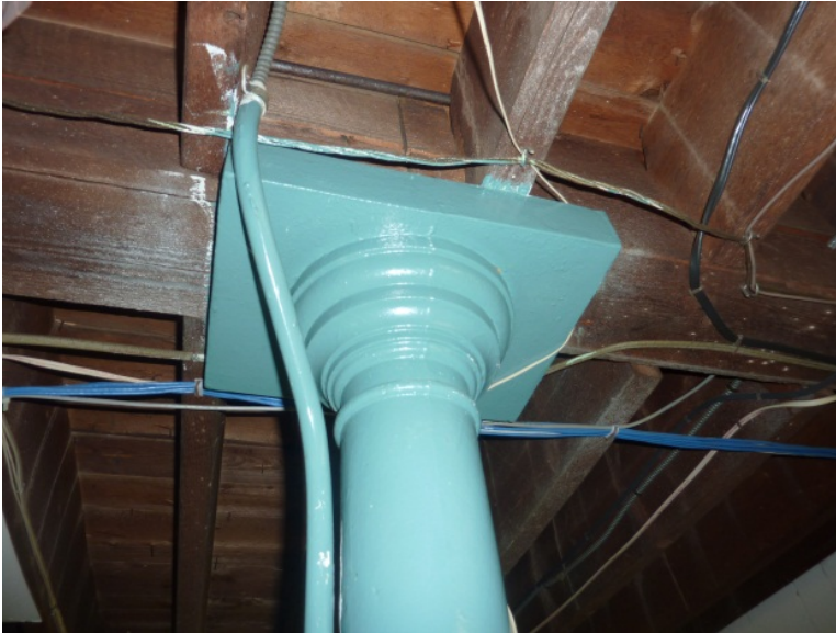
Cast iron column capital at basement supporting first floor framing.
