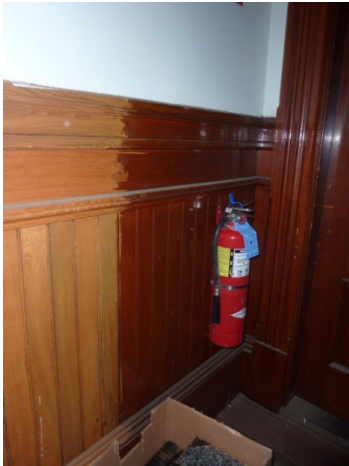
Original dark stain and varnish has been striped to reveal color of original wood at attic level.
