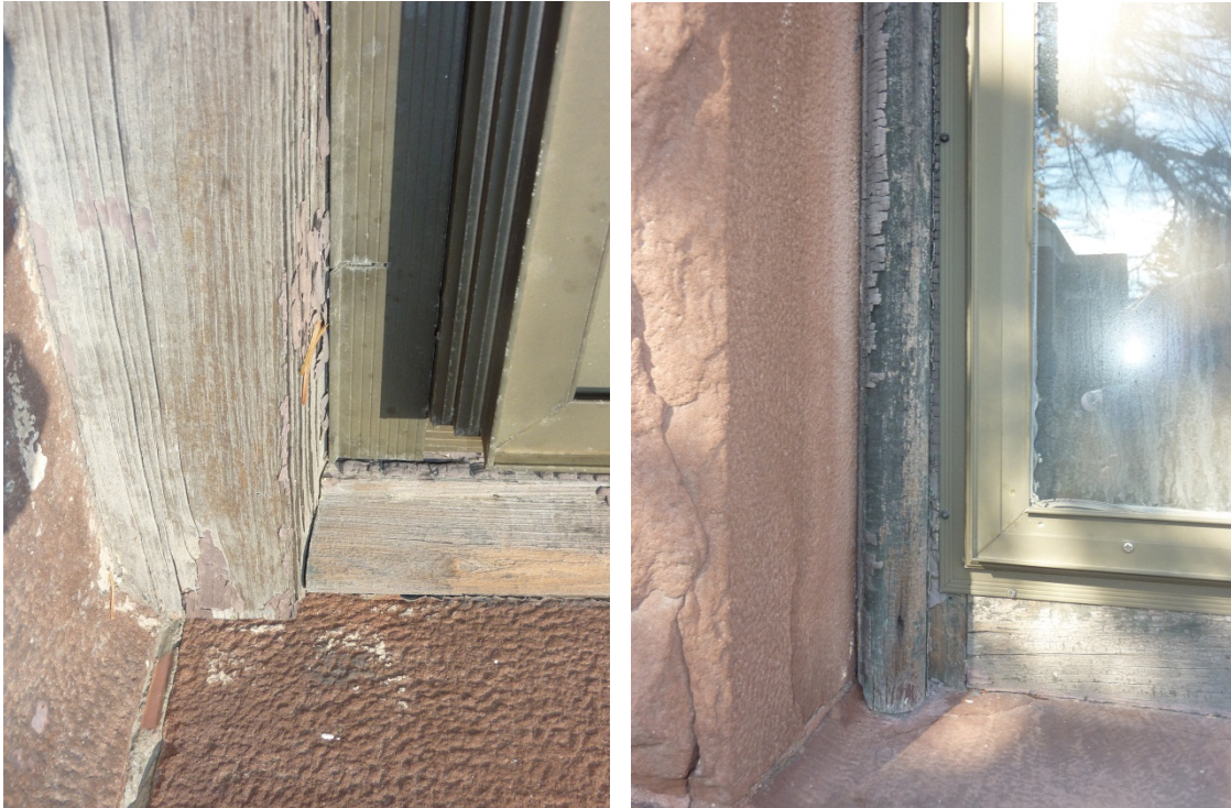
Exposed wood exterior trim with storm window screwed to wood frame.
