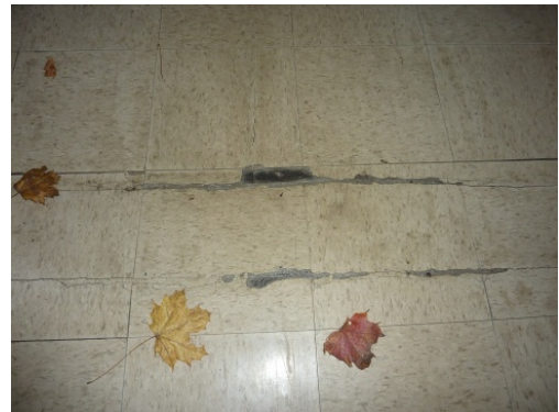
Vinyl tile on wood framing in offices and restroom
