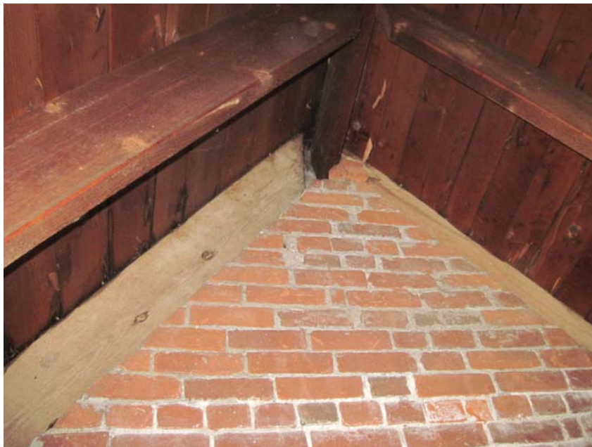
Figure 4: Ridge at Gable Wall
