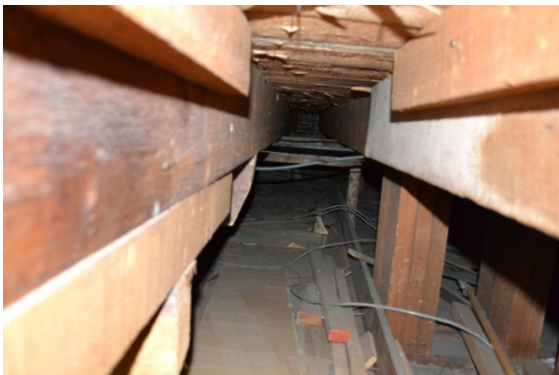
Framing of stage and second floor framing runs to exterior walls.
