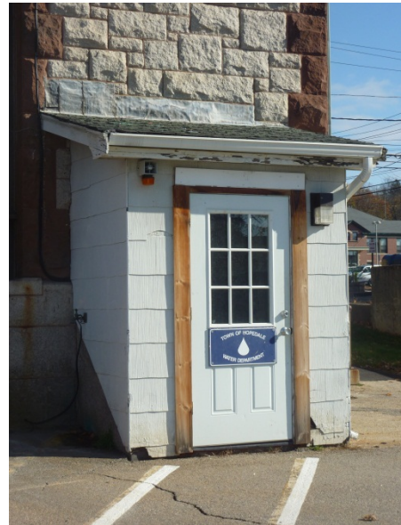
Exterior door at south basement entrance.
