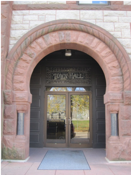
Exterior doors at main entry.
