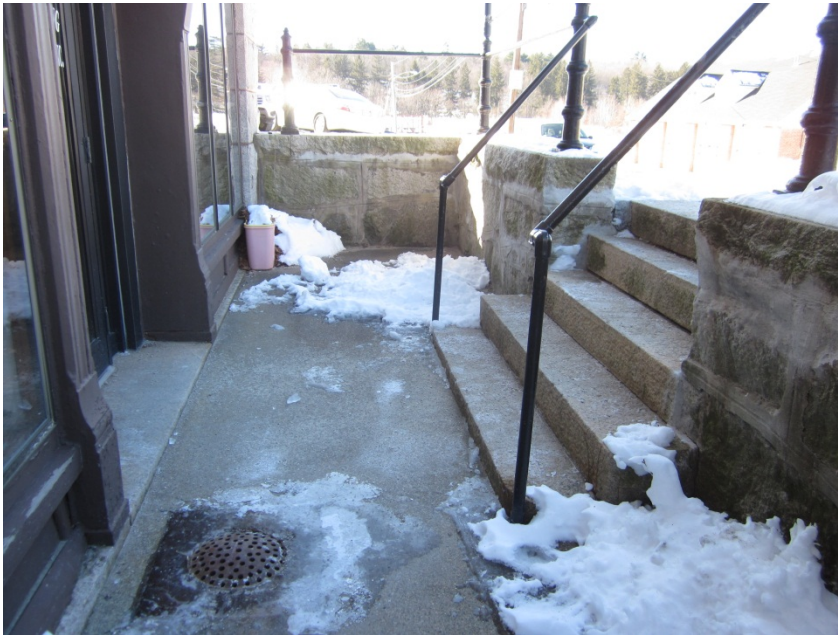
West basement entrance to the Council on Aging Shop.
