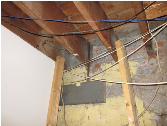
Wood first floor joists at exterior wall.
