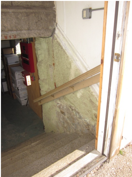
Stair to basement from parking lot.
