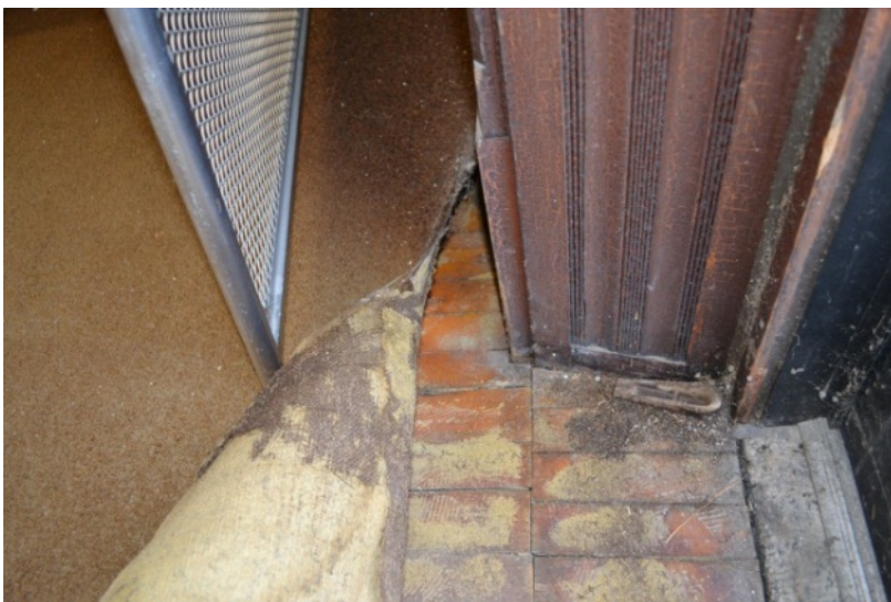
Wood flooring at auditorium under existing carpet
