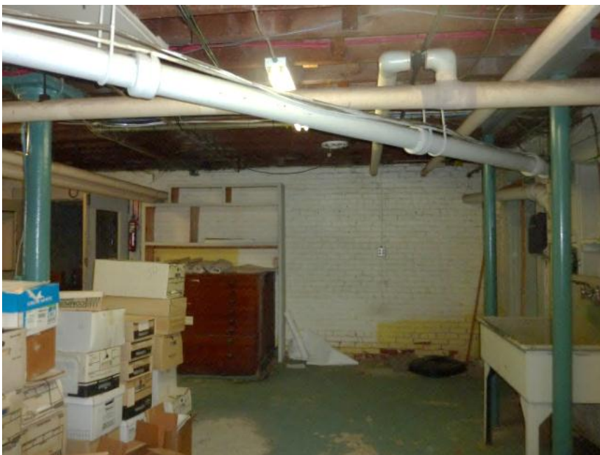
Brick load-bearing interior partition wall in northeast storage room.
