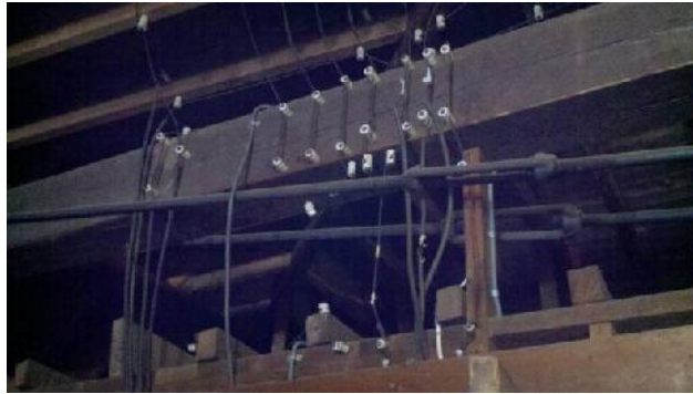
Figure 7 - Knob & Tube Wiring
