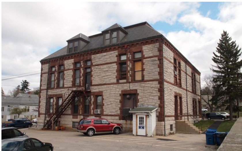
Southeast view of Hopedale Town Hall.
