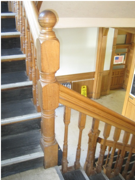
Wood corner post at landing of first and second floor.
