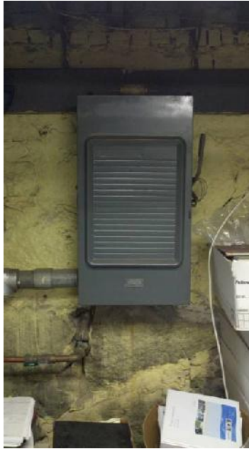
Figure 6 - Service Disconnect
