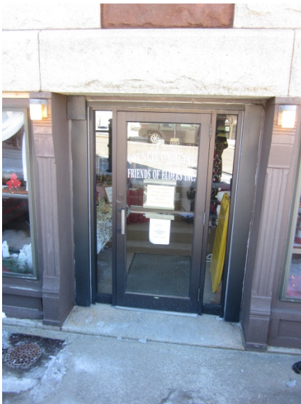
Exterior storefront door at Council on Aging.
