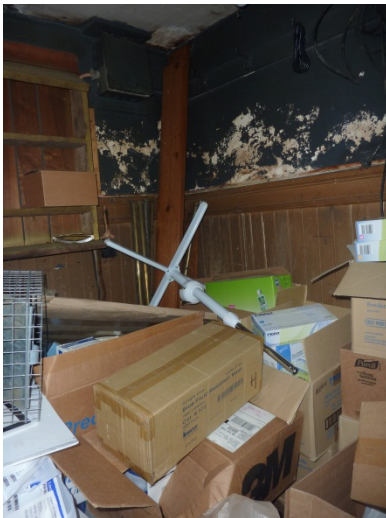
Original beadboard and plaster in Heath department office closet.
