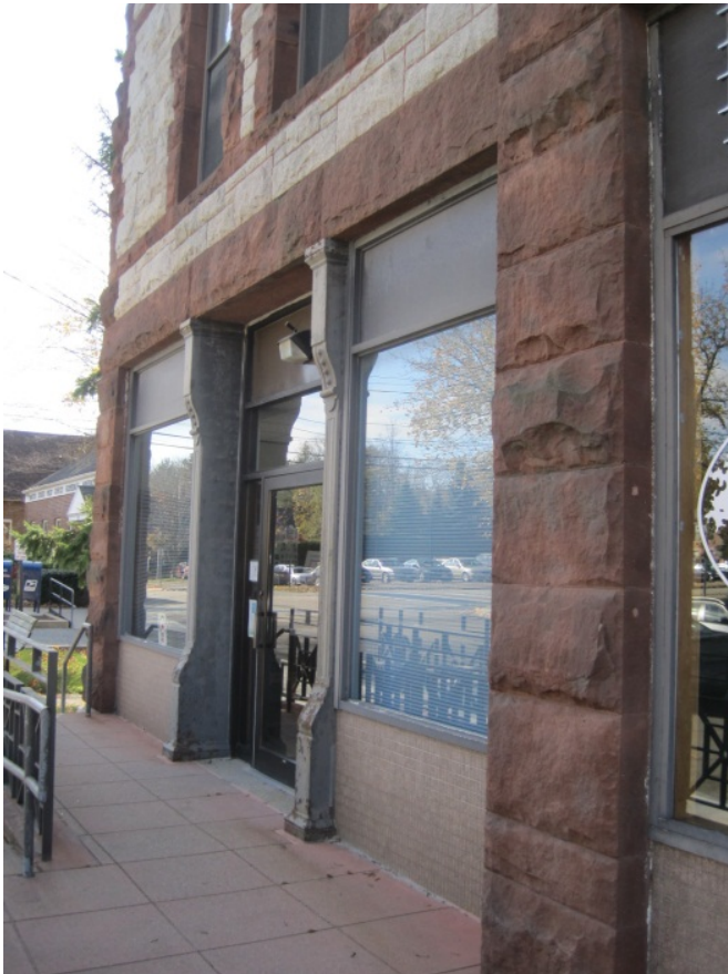
Aluminum storefront windows at north elevation.
