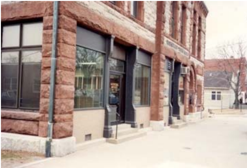
Exterior plaza at north elevation in 1989. Note the stone steps and base of wall and pilasters visible. (www.robertnicholsdesign.com)
