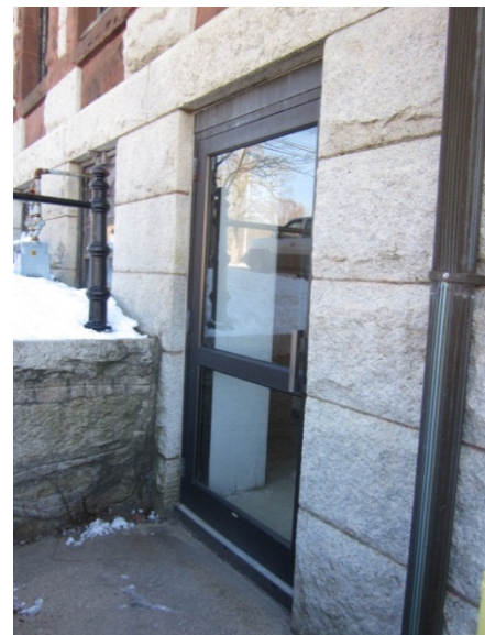
Exterior door at basement office area.
