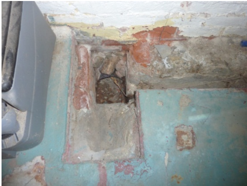
Trough at northeast storage floor.
