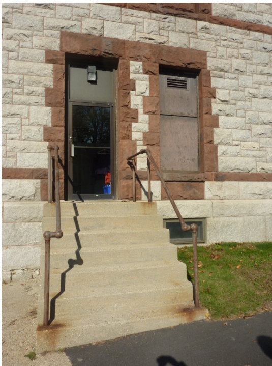
Concrete stairs at east elevation.
