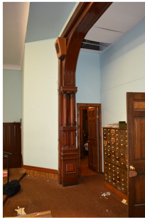
Wood stud partition at stage with elaborate wood casing
