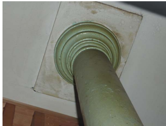
Cast iron column capital at first floor supporting second floor framing.
