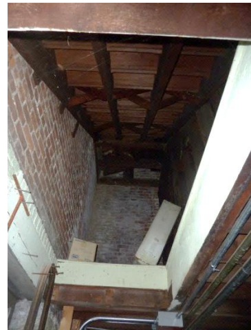
Location of a former stair to the basement.
