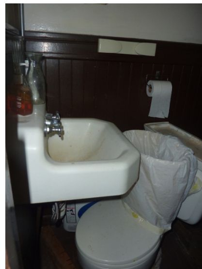
Second floor abandoned restroom
