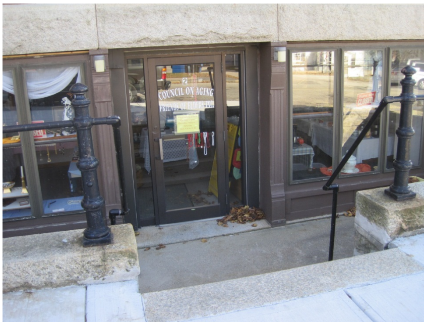
Original wood framed storefront windows at Council on Aging basement entrance.
