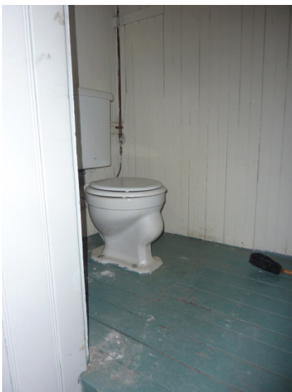
Basement abandoned restroom
