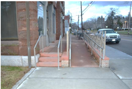
Stair and ramp at east elevation
