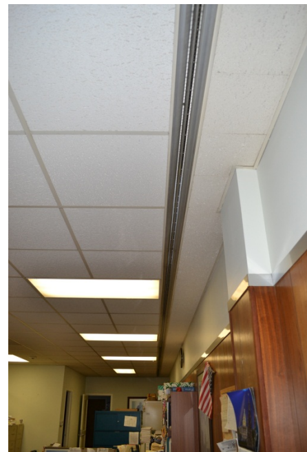
Acoustical ceiling tile at general office
