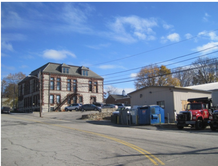
View from Depot Street looking northeast.
