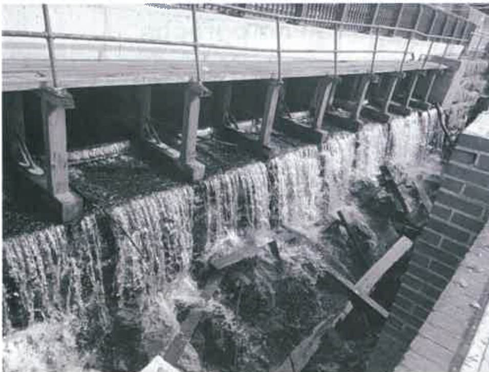
Photo 2 – Overview of spillway from downstream showing existing catwalk
