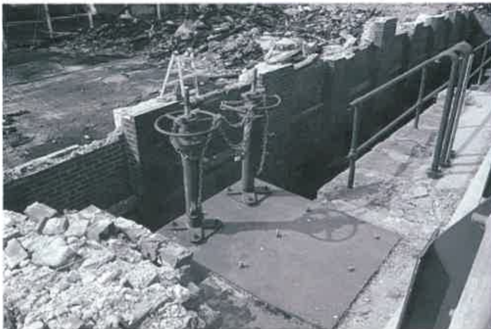
Photo 6 – left sluice gate operators
