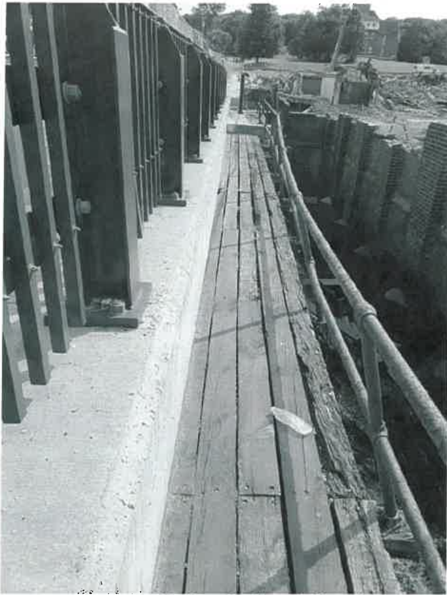
Photo 7 – Existing catwalk and sidewalk
