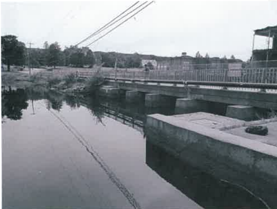
Photo 1 – Overview of bridge and dam from upstream
