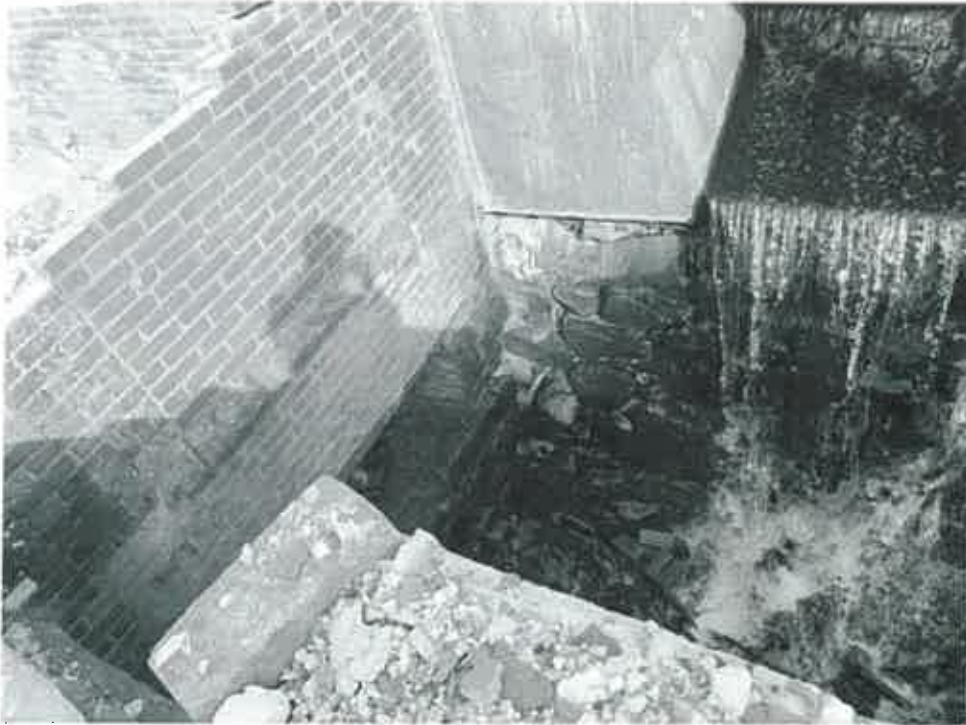
Photo 3 – Right end of spillway weir and bridge abutment from downstream
