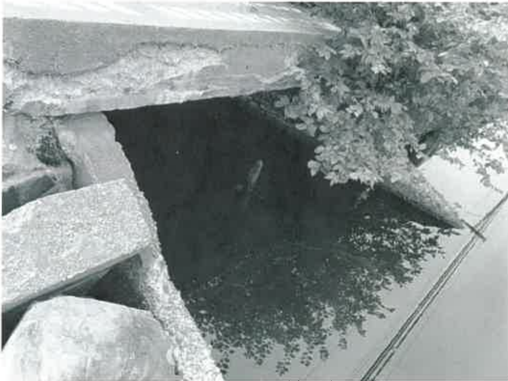
Photo 11 - Left outlet inlet
