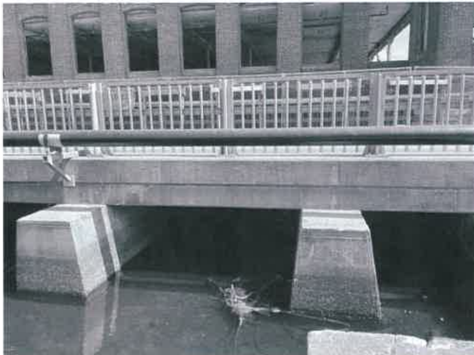
Photo 9 – Bridge from upstream, showing one opening and gas main
