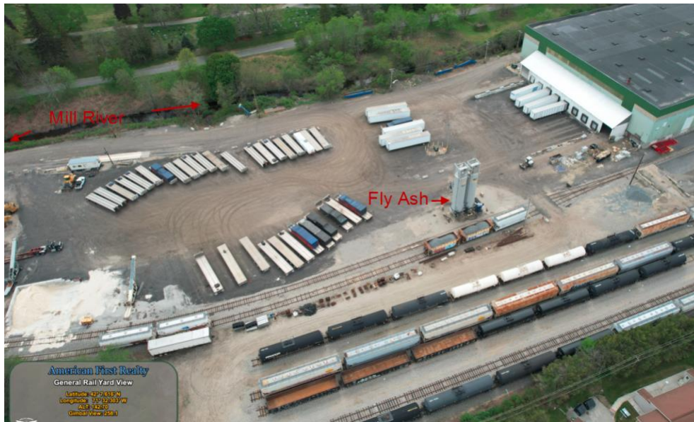
Front portion of the railyard showing fly ash storage (May 2022)
