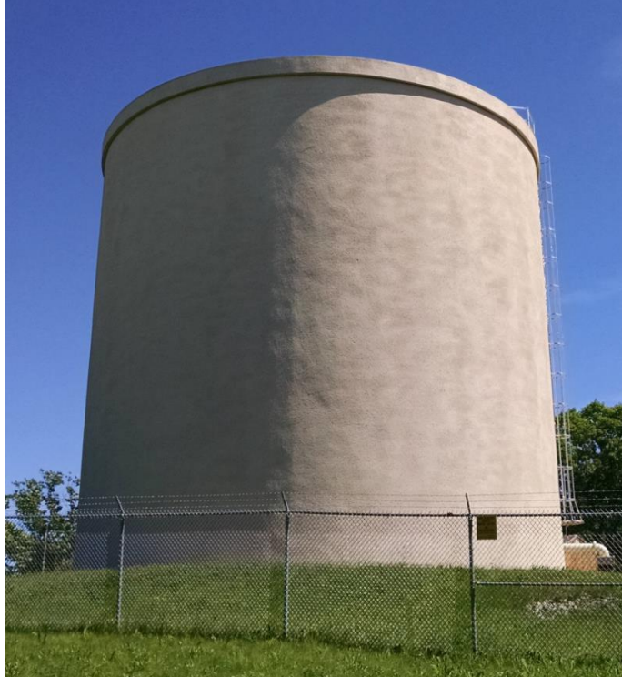
Figure 3: Weston & Sampson prestressed concrete standpipe tank project.
