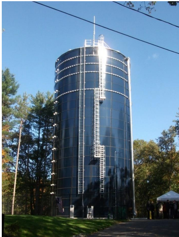
Figure 2: Weston & Sampson GFS standpipe tank project.
